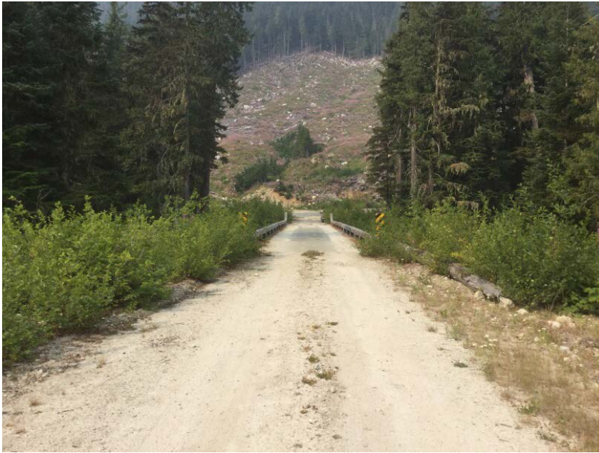
Approach from Right Bank when facing downstream
