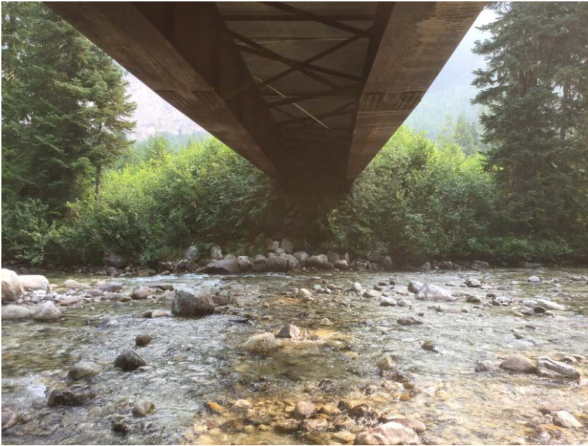
Right Bank Abutment when facing downstream
