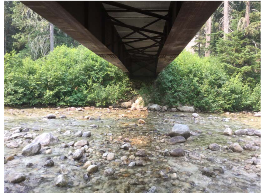
Left Bank Abutment when facing downstream
